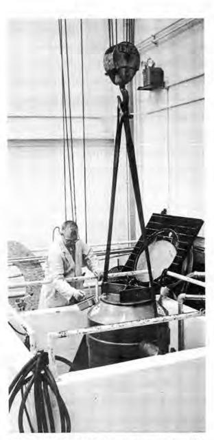
SPECIAL SHIPPING CASK containing four fuel elements from Sandia Engineering Reactor is raised for radiation readings by Health Physicist Charles Berglund (3311). Work is being done in connection with final shutdown of reactor after many years of service.
